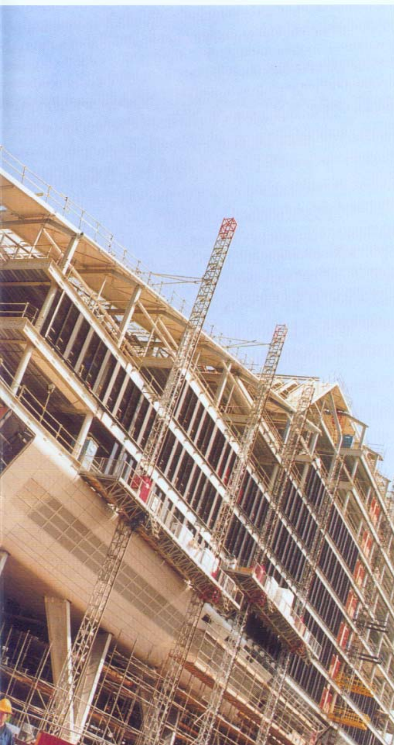
Basic mast climbing work platform Extension
