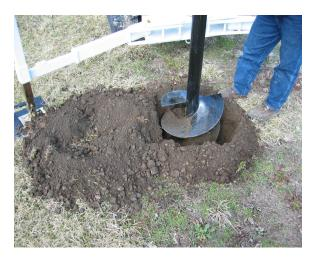
If needed, an extension bar may be added to reach proper depth.
